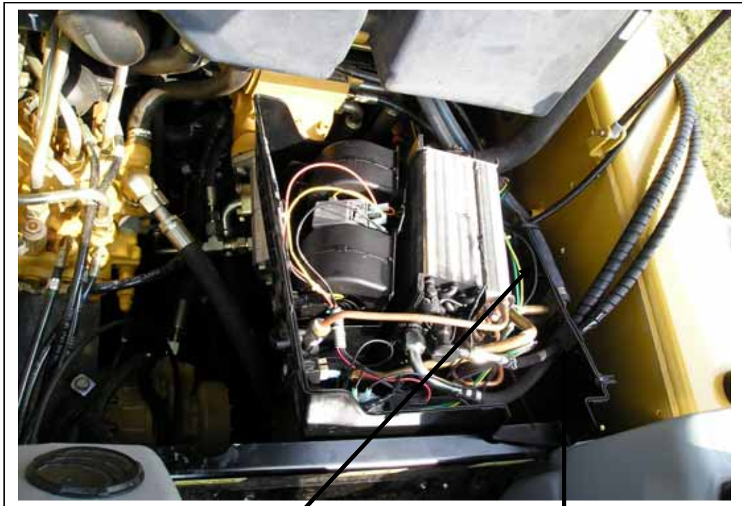
Relay control wire exists with other wiring
